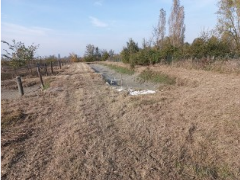
5.II° grid at the point of water discharge
