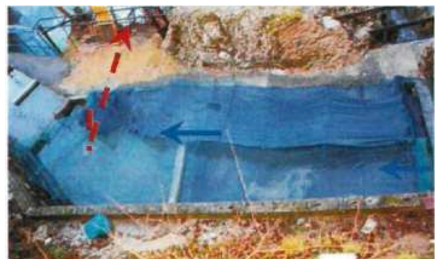
The second and third raceways receive the waters from one of the three swing pipes and discharge into the torrent through independent pipe with regulator pipe
