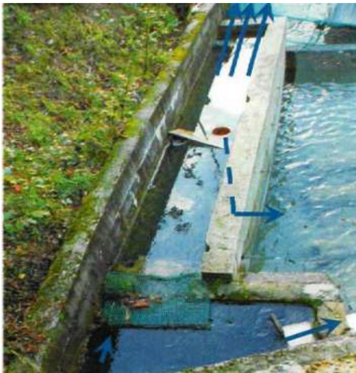
The plant is fed by the waters of the Nossana torrent, which are derived in a loading basin from which the distribution branches off. There are five exits from the basin: one at the top of the free surface feeds the first concrete basin; a central unit (overflow and regulator) which again flows into the first tank; three swing pipes that feed the second concrete tank (and the other five in series), the internal tanks and incubators.
