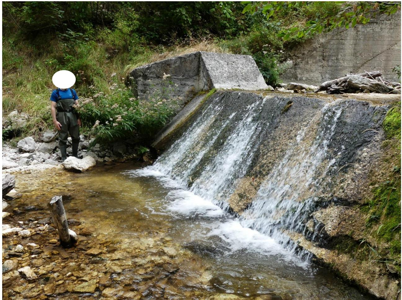
Figure 3: Barrier which prevent the upstream movement of aquatic animals into the zone Tenna. Upstream side (coordinates: 42° 55.307'N - 13° 16.755'E).
